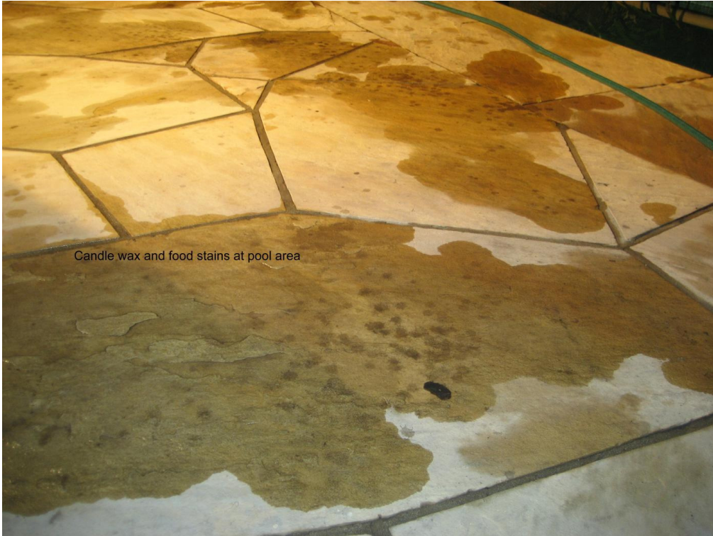
Before and after removal of wax and food stains from Sandstone
