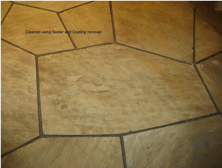
Before and after removal of wax and food stains from Sandstone
