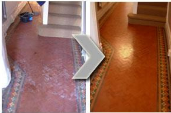
Before and after restoring terracotta tiles.
